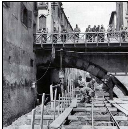
The bridge during the enclosure of the waterway
